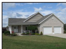
Finished home in Adams County
